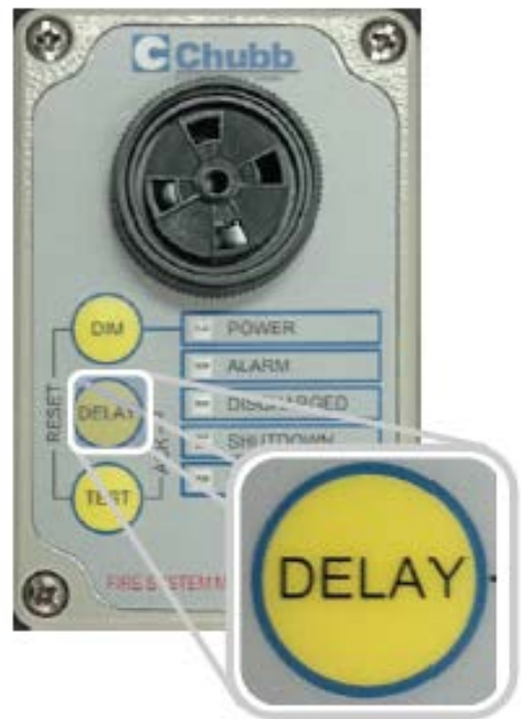
Figure 9 - Shutdown delay button
