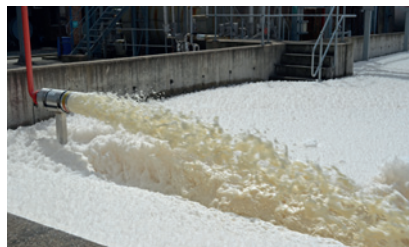
MEX Bund Pourer in action
