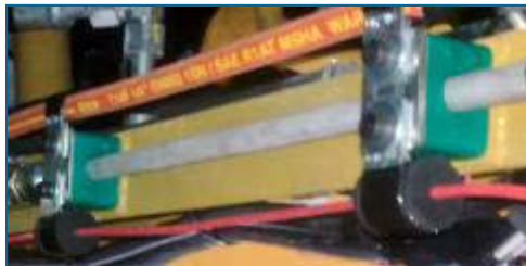
Figure 58 - LHD cable installed
